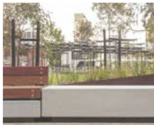
Timber clad concrete planter beds
