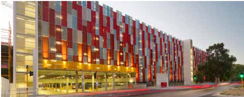
EXISTING MULTI-DECK CARPARK AT QEIMC
