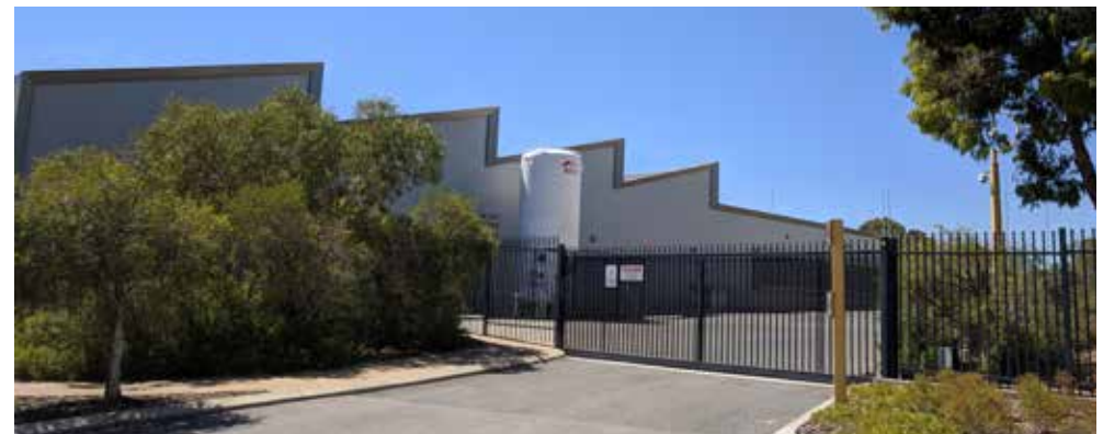
SECURE SERVICE ACCESS AREA
