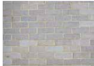
Brick paving from site
