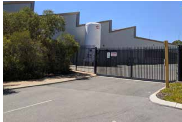
Example of back-of-house / service road within Campus.
