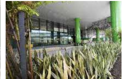
UNDERCOVER DROP OFF AREA
