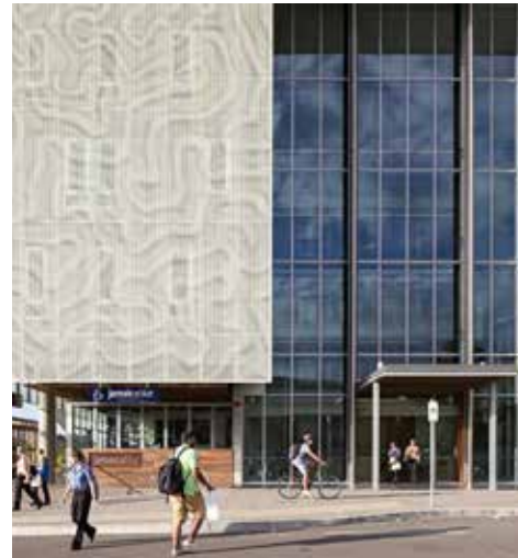
FACADE SUN SHADING
