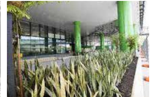
UNDERCOVER DROP OFF AREA
