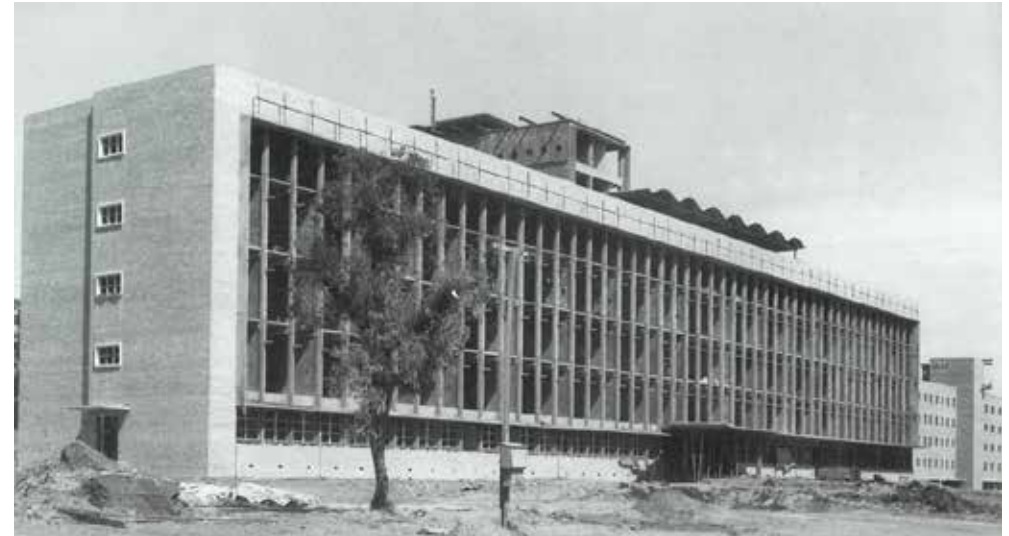
Perth Chest Hospital under construction with nurses' quarters (right) early 1958.
