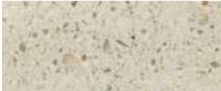
Exposed aggregate concrete
